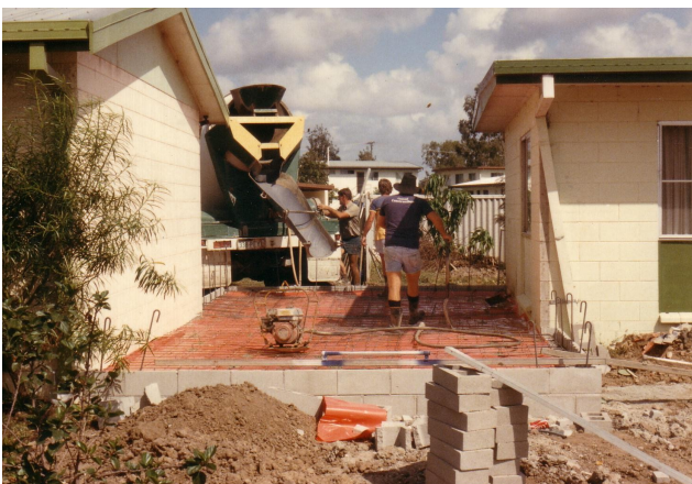
Laying the slab for the office extension, viewed from the road. HAIGPHOTO
